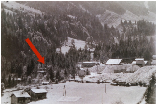
Fig. 1 1940s photo of Suggadin camp (red arrow) and the construction site of the water bridge (foreground; image: LAV).
